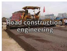
Road Construction Engineering
